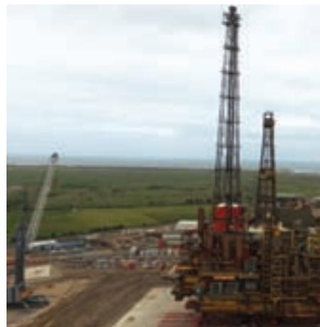
Solmek supervision, using a Symmetrix drill string to advance the boreholes through made ground and drift deposits using air as a flushing medium.
